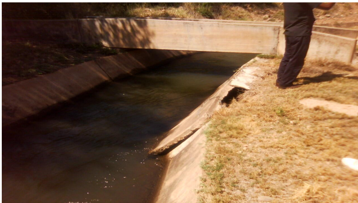
Photo 5.2: Major Cracks on the N canal in the joints of the concrete panels
