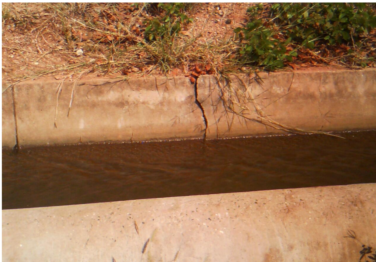
Photo 8.1: Broken section of concrete panels of canal system
