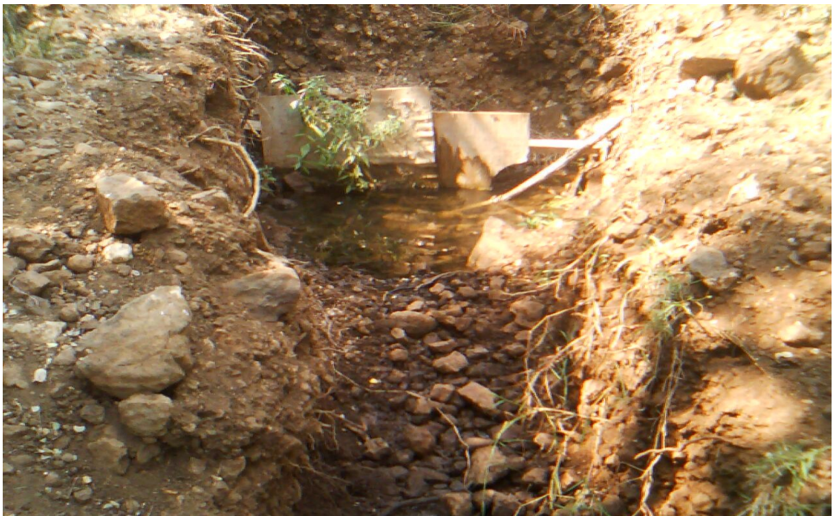
Photo 5.9: Leakage on the canal siphon as a result of the algae infested canal
