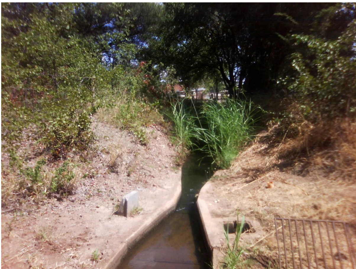
Photo 11.1: Sluice A8 suspected of submerged flow conditions
