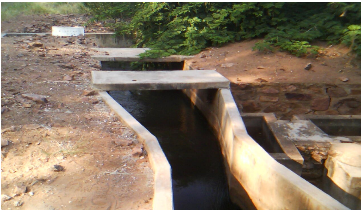
Photo 4.1: Flow measurement at the inlet to the A canal siphon on the Nzhelele River canal system
