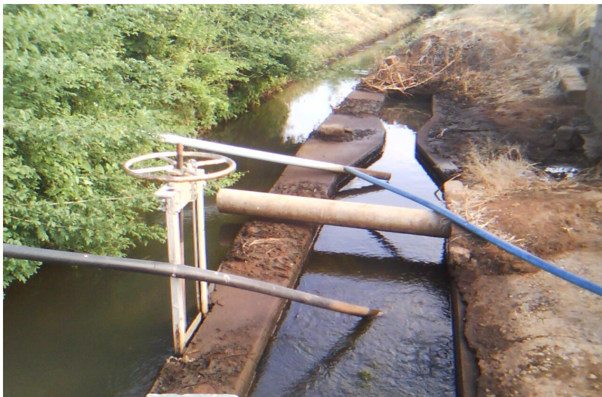
Photo 10.2: Submerged Parshall Flume on the A branch canal with no visible hydraulic jump at the throat
