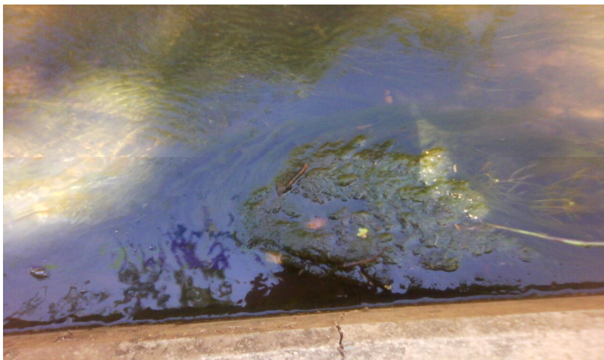
Photo 8.2: Aquatic weeds and algae in the Nzhelele Irrigation Canals
