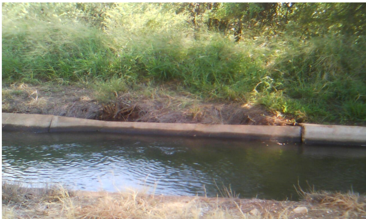
Photo 5.1: Open joints between the concrete panels as well as growth in the canal
