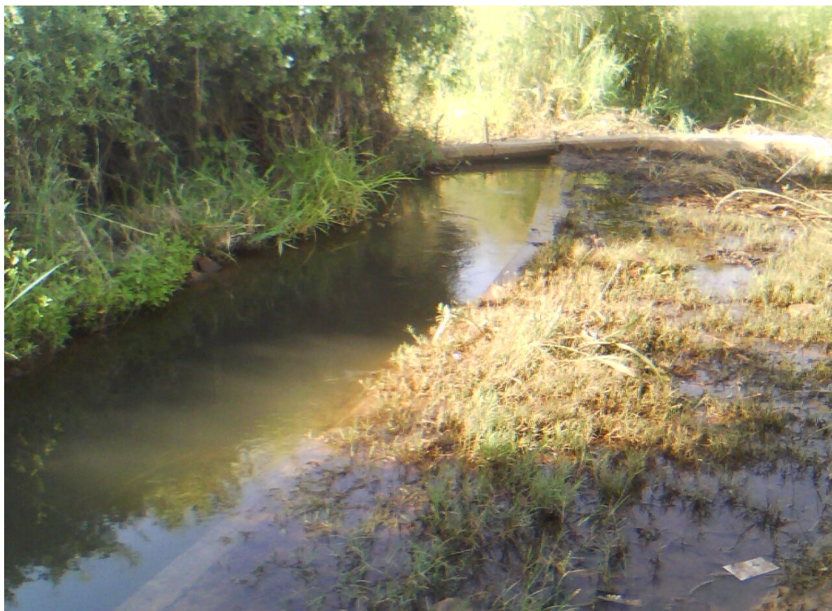
Photo 5.7: A branch canal overtopping as a result of the algae growth in the canal
