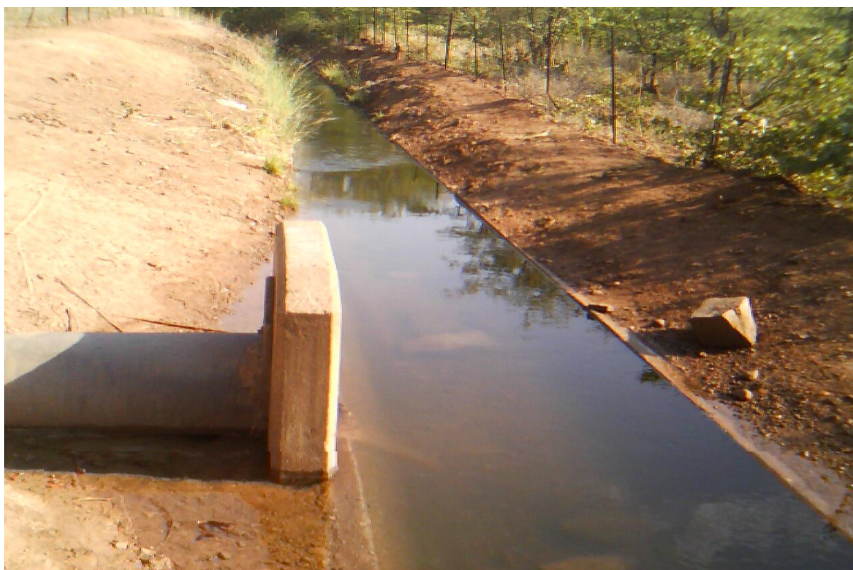
Photo 10.1: Overtopping in the A branch canal due to aquatic weeds and excessive irrigation water as upstream irrigator does not pump the full order
